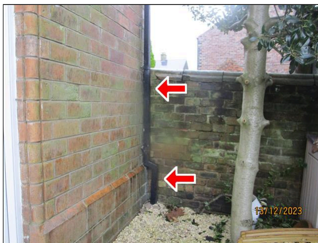
7.2 Item 2(Picture) Boundary wall abutts main wall
