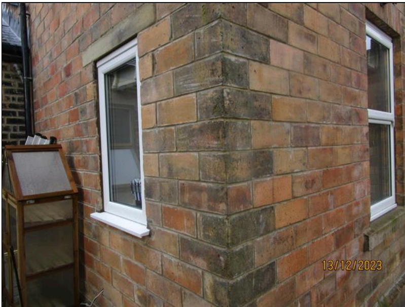
7.0 Item 1(Picture) Stone wall construction to main walls
