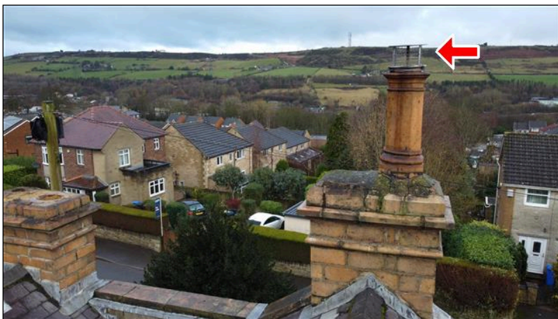
4.2 Item 3(Picture) Chimney with cowl
