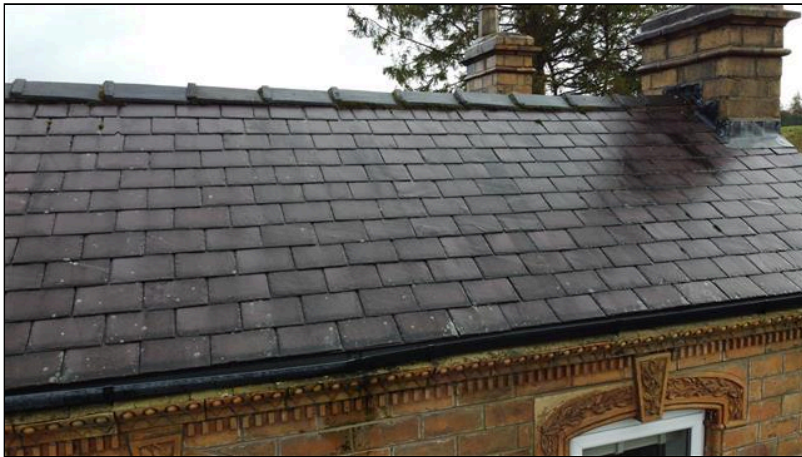
5.2 Item 2(Picture) Rear elevation roof
