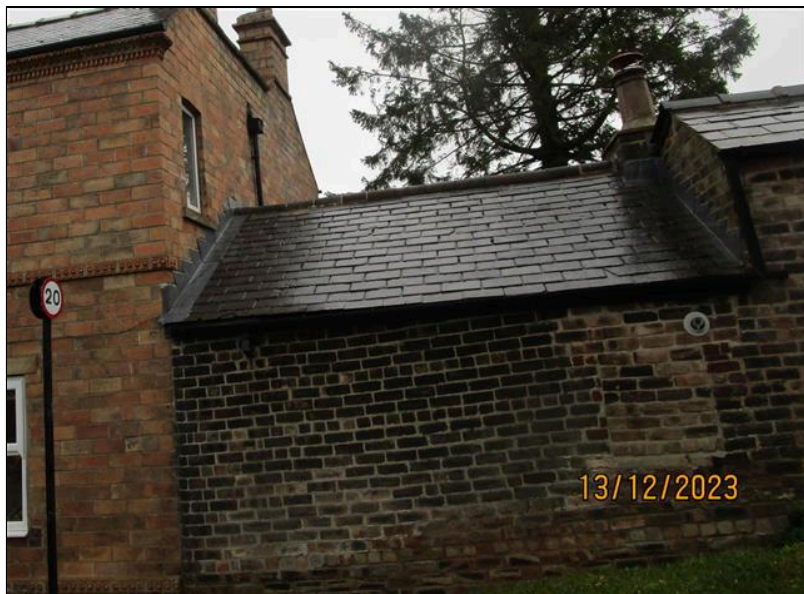
7.0 Item 2(Picture) Single brick walls to the Utility Room
