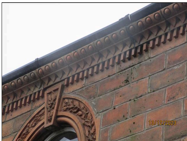
7.2 Item 3(Picture) Walls recently repointed
