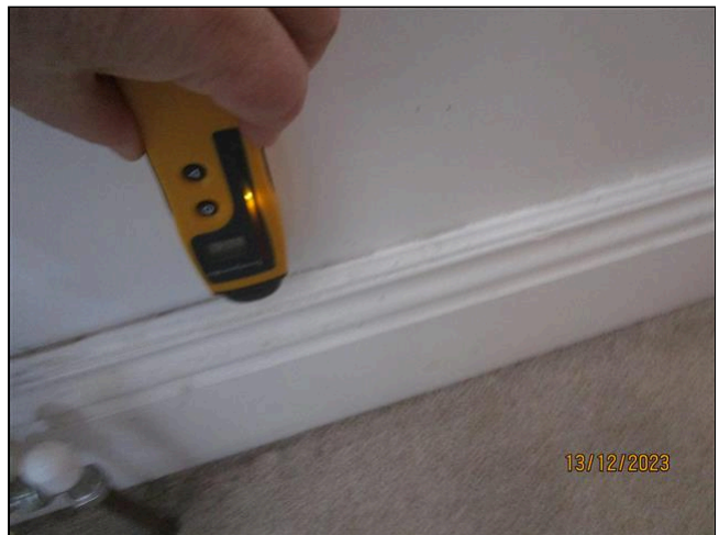
3.0 Item 4(Picture) Damp check with moisture meter
